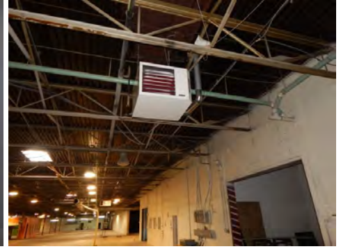
Multiple overhead heaters various ages and brands
